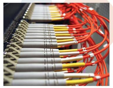
Fibre optic cabling provides greater bandwidth than copper ensuring faster speeds at which data can travel. It has increased security and zero electromagnetic noise and interference which means it is more reliable.
